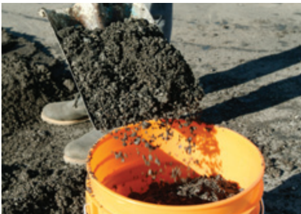
IMAGE A: Milled asphalt containing GlasGrid product can be easily recycled for use on other projects.
