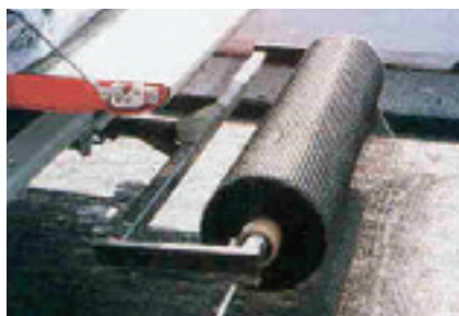
IMAGE L: Manual placement of the GlasGrid System.
