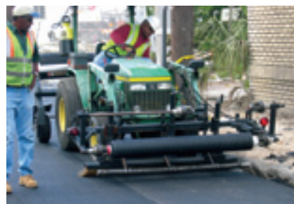
IMAGE M: Overlapping the GlasGrid System across transverse or longitudinal joint.
